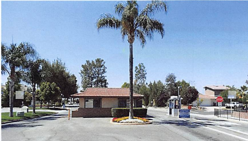
Learn at next week's POA Board meeting if and when the Main Gate Project is set to begin. Photo by Donna Kupke.
